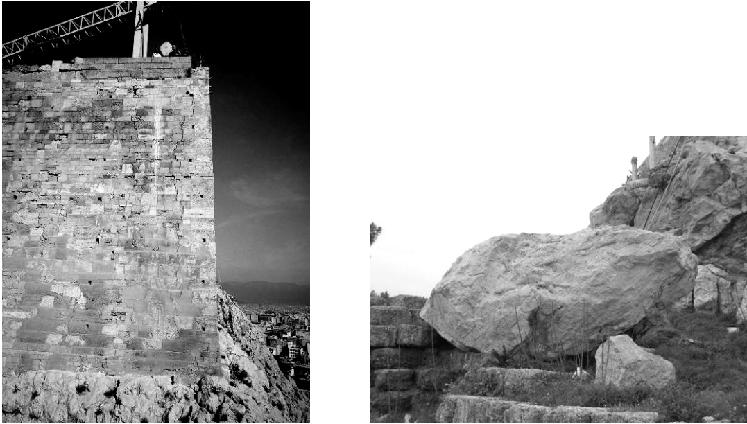
Figure 2. Left: Recent photo of the SE side of the SE/E part of the Acropolis Wall in Athens. The fissures on it are apparent. Right: Sizeable detached rock block of the SE/E part of the Acropolis Hill in Athens
